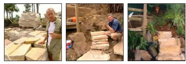
Blitz tipz: Yellow brickies sand and off-white cement makes a good colour match to most sandstone.
