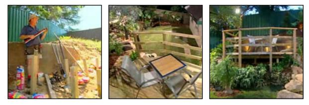
**Daybed:** Jamie builds his deck using the same posts (90x90mm) in ground and bearers (140x45mm) but does not need to use joists because he uses timber 140x45mm H4 treated that can span his bearers.
