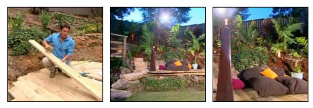
**Paving:** After inspection of existing pavers, which were found to be stable, Nigel decided to pave directly over old pavers with a large format paver. Preparation for this process is the same as if laying over a roadbase or over concrete. Screeding sand was used to achieve levels. Pavers were then laid in the usual way making sure that all ends were locked in by haunching with a mix of 4:1 sand to cement.
